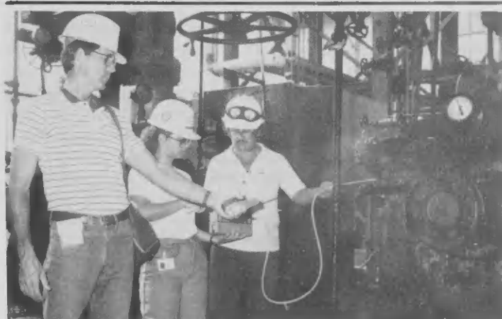
William Smith of Exxon's Research Environmental Health Control along with Rusette Arends and Simon Geerman of Lago's Safety Section are checking for hydrocarbon gasses at a leaking pump, during the two-week annual Environmental Health Control.
